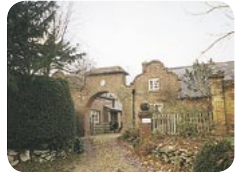
Gateway pier to former Ellisfield Manor
